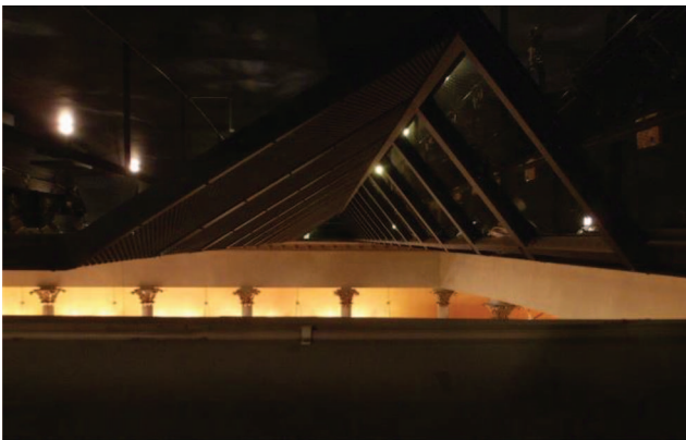
Figure 2. Acoustically semitransparent metal mesh ceiling, partly horizontal (far left and far right), partly angled in section (center left) in order to reveal lighting bridges (center right). The semitransparent metal mesh ceiling creates a transmission loss between the main acoustic volume of the hall and the volume below the ceiling. See the online article for the color version of this figure.
